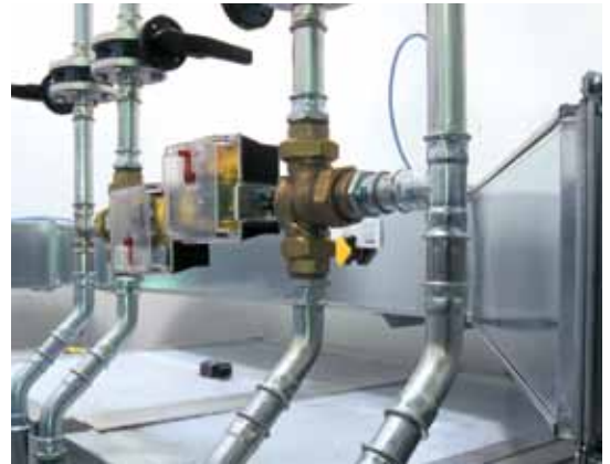
Figure 22 - Steelpres - refrigeration circuit
