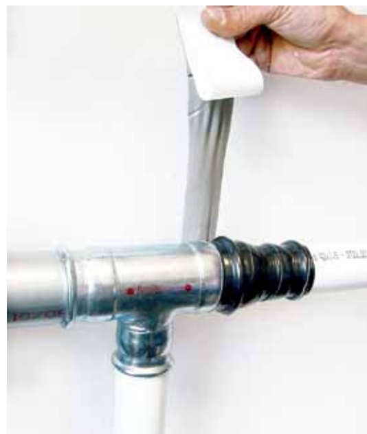
Figura 35 - Protection of the connectors with butanol adhesive tape
