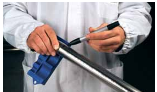
Figure 28 - Marking the insertion depth
