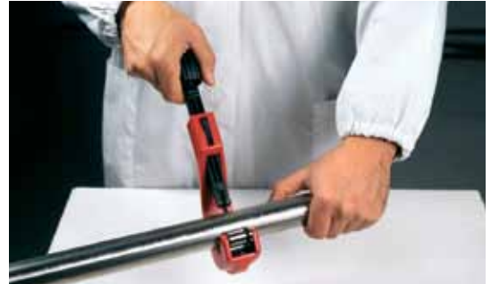
Figure 25 - Cutting the pipe to length
