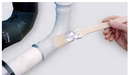
Figure 34 - Varnish of the connections and pipes with primer.
