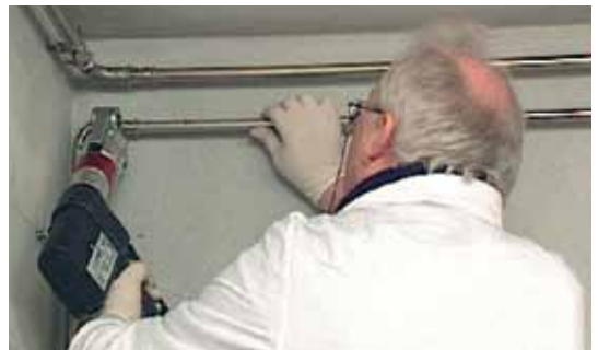
Figure 32 - Making the press connection
